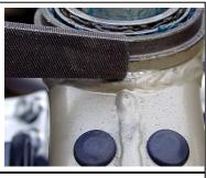
Using a sharp file, start at the high spots and trial fit the bracket until it fits properly.
