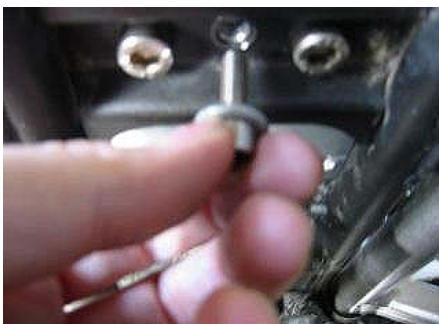
Bottom riser bolt with washer installed
